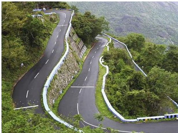
(This road has excessive cuts and does not follow the natural contour of the land.)
