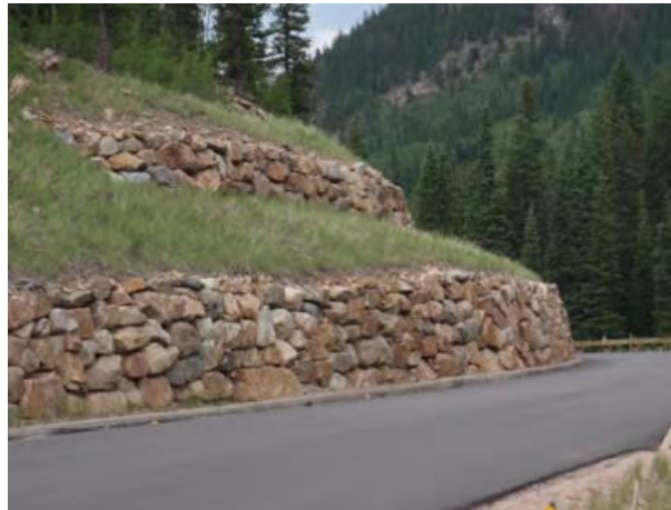
(Retaining wall faced with stone. Terraces have been revegetated.)
