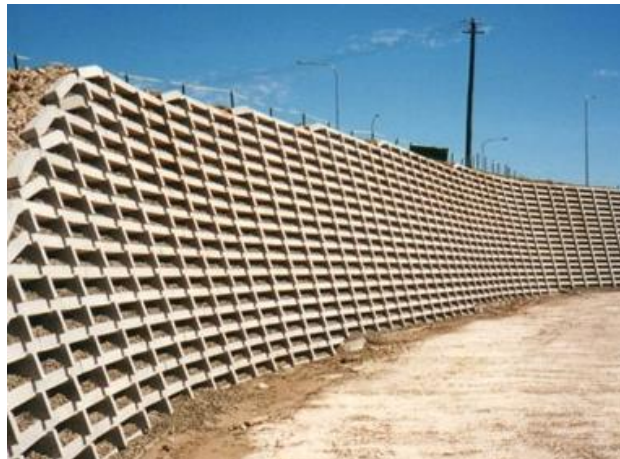
(Wall is not constructed of earth-colored materials and does not provide opportunities for planting pockets.)
