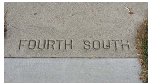
Figure 4.1 - Stamped concrete wayfinding
