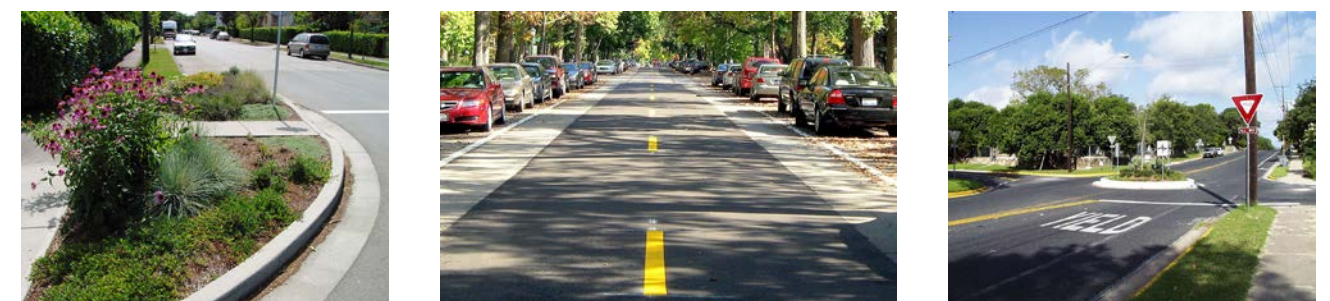
Figure 4.7 - Traffic calming strategies for Franklin Neighborhood city streets (bulb-out, striping, traffic circle)
