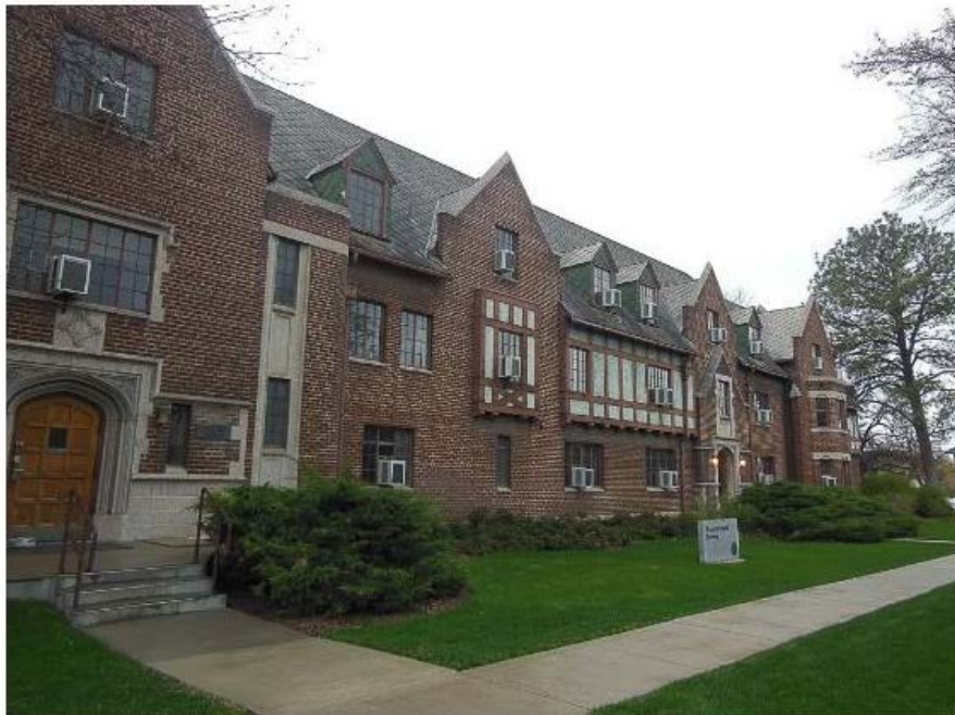
Photograph 2 North elevation. Camera facing southwest.
