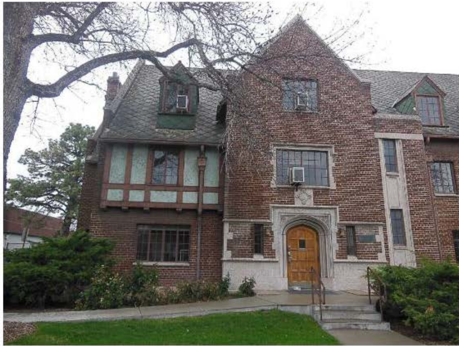
Photograph 3 East end of north elevation. Camera facing south.
