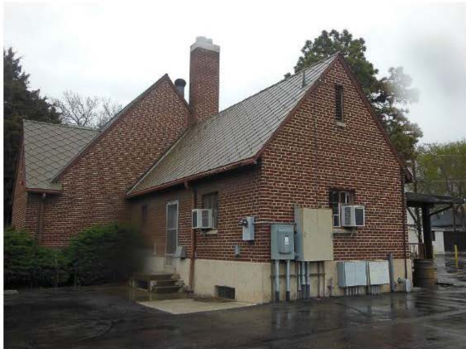
Photograph 6 South and west elevations of kitchen wing. Camera facing northeast.
