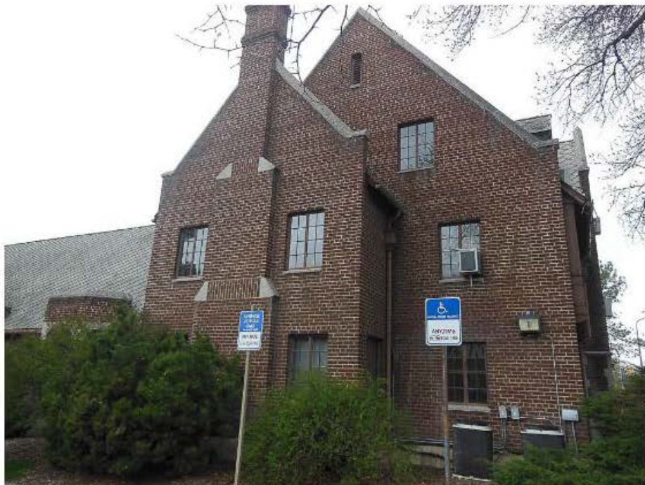
Photograph 4 North end of east elevation. Camera facing west.
