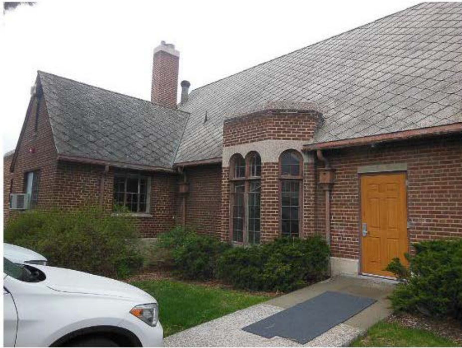
Photograph 5 East elevation of dining hall & kitchen wing. Camera facing southwest.
