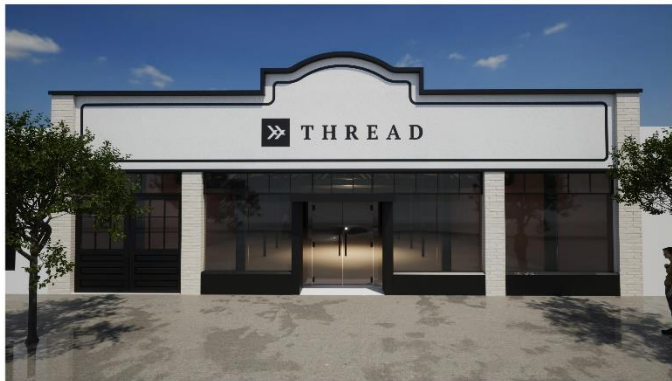
3 CENTER STREET FACADE VIEW LOOKING SOUTH
