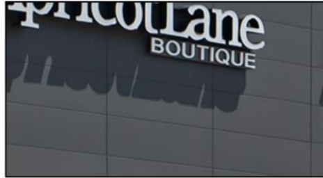
ARCHITECTURAL FIBER CEMENT BRICK SIDING - BRK-1 BRAND: NICHIIHA COLOR: STEELE FINISH: TUFFBLOCK
