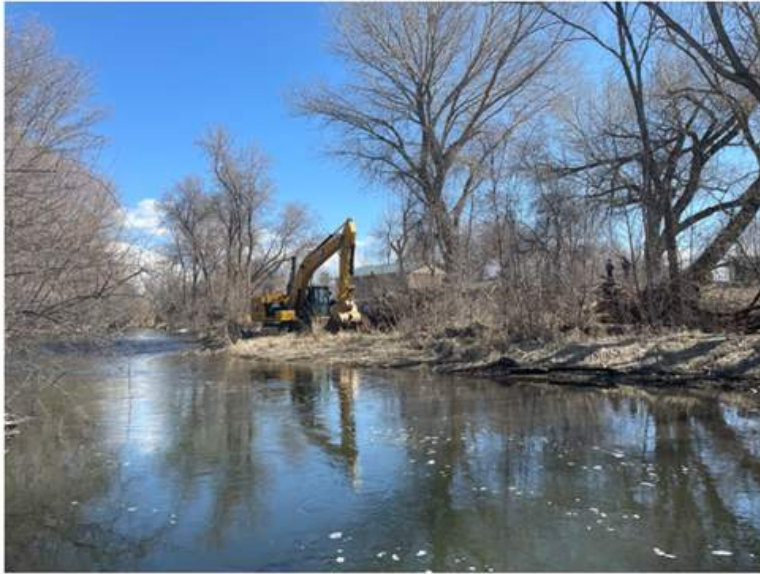
Provo City Public Works crews clear away debris from the edge of Provo River. By reducing the debris along the edges of the riverbed, the city will allow water to flow easily through the floodway and avoid surging up into residential and commercial housing. (Photo courtesy of the city of Provo)
